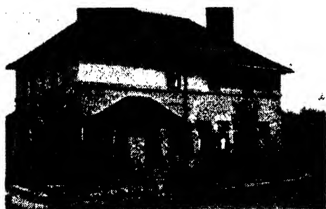
Photograph of Building Cured by "BETEX"
