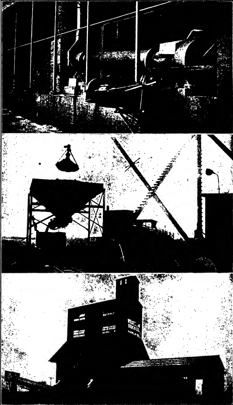
FIG. 4-10.—Views of Haydite manufacturing plant. Top , kiln and clinker conveyor. Center , handling from storage pile to loading chute. Bottom , grinding plant.
