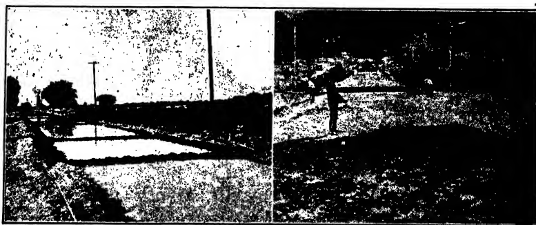
Left, ponding. Right, covering with dirt and wetting intermittently.
