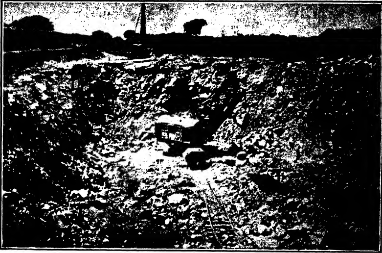
FIG. 2-1.—General view in stone quarry from which limestone is secured.
