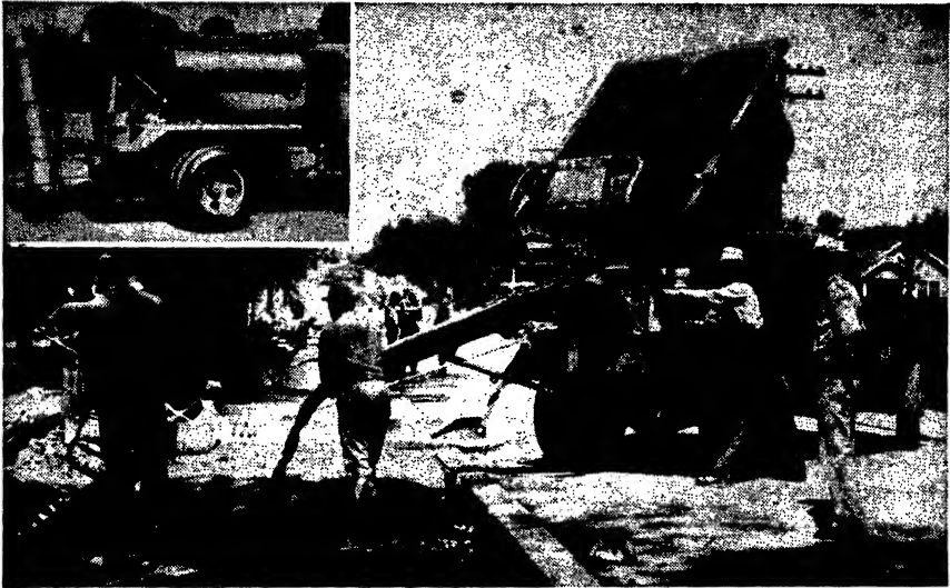
FIG. 9-1.—Concrete being discharged from a truck body, known as Dumpcrete, on a pavement-widening job in Tulsa, Okla. This truck body was designed primarily to haul air-entrained ready-mixed concrete without agitation. The high dumping position permits concrete to be chuted into wall or slab forms, or into concrete buckets or buggies. It is not necessary for the truck to operate on the subgrade between forms on paving work. Bodies are made to handle 2, 3, or 4 cu. yd. of concrete. Insert, body in the horizontal, hauling position. (Mazon Construction Co., Inc.)
