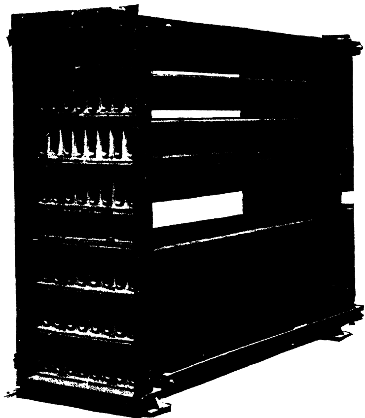
FIG. 34. GREEN'S OVAL TUBE AIR PREHEATER (E. Green & Son, Wakefield)
