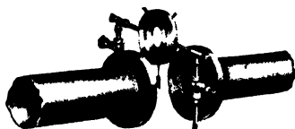
FIG. 102. CARRIER RING ORIFICE PLATE AND FITTING ( Electrofto Meters, Park Royal )
