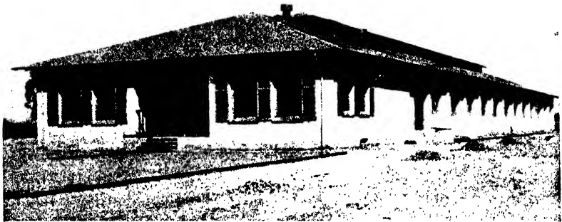
FIG. 132.—The new Los Angeles County Insectary built at Riviera in 1929. It is a splendid modern semifireproof building 200 feet long and containing 24 production rooms, each 12 x 18 x 8 feet and each with a capacity of 360 trays of host plant material and a productive capacity of approximately 150,000 ladybird beetles each five-months period. In the front are office and laboratory rooms. (Photograph and information furnished by H. M. Armitage, the superintendent.)
