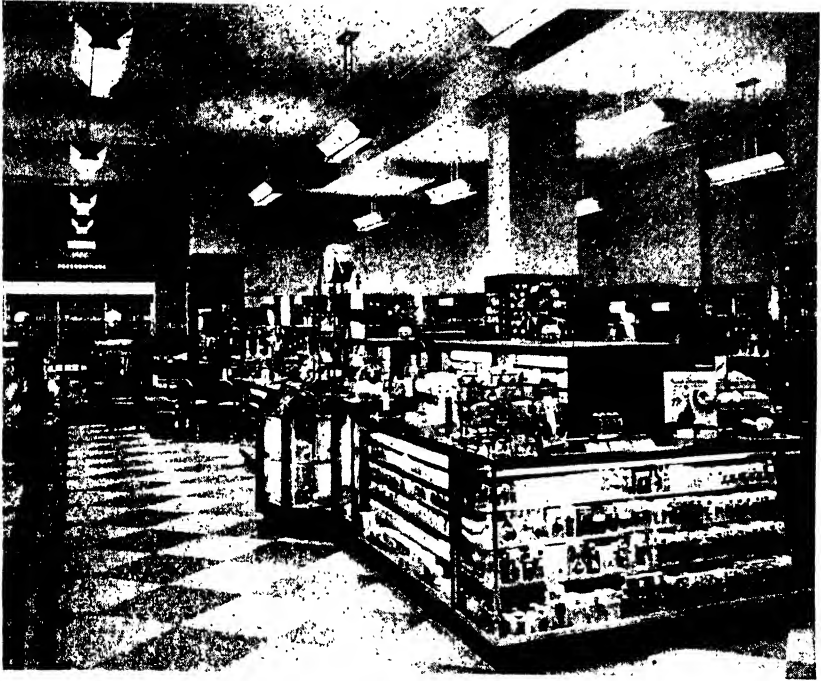
Fig. 11. Fluorescent lighting in individual units (Liggett Drug Company, New York City). This installation uses 68 forty-watt units to illuminate 2,112 square feet of floor area—a room 44 by 48 feet. The wattage is 1.28 per square foot. (Courtesy of General Electric Company.)
