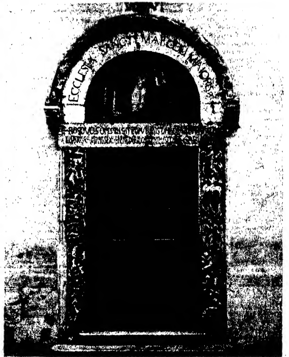
FIG. (B), above.—Pisa Cathedral. Opening 11 ft. 6 in. wide. White, gray, and buff marble. Marked Classical influence. (Fig. 261 B)
