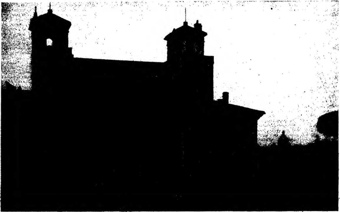
FIG. (A), above.—Duality created by presence of two equally dominant towers. Lack of unity. S. Sulpice, Paris.
