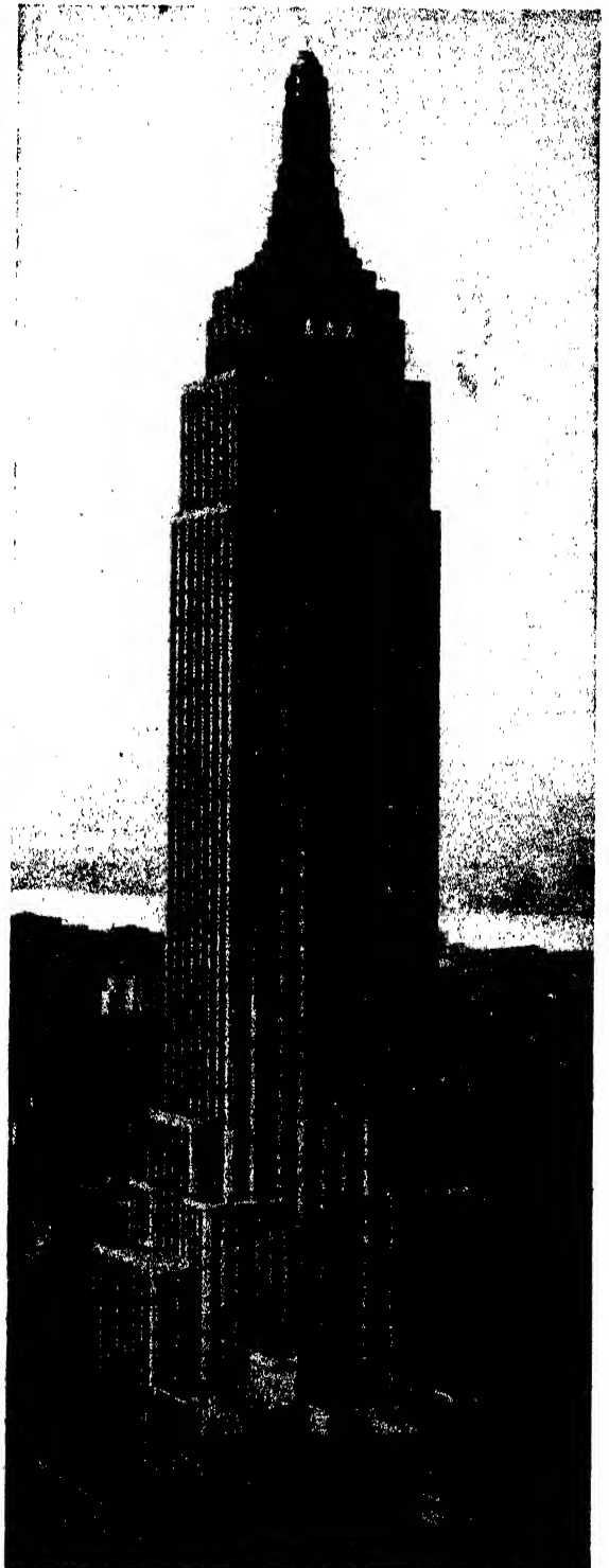
FIG. (A), left.—A study by E. Saarinen for Chicago Tribune. Early application of vertical, set-back principle of design and construction. FIG. (B), right.—Ten years later than (A). The ultimate expression of soaring verticality. Limestone and steel. Empire State Bldg., N. Y.
