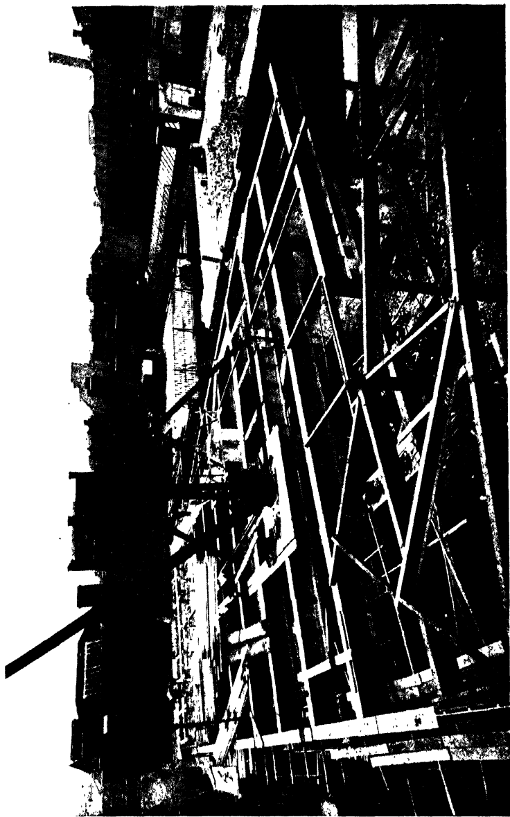
FIG. 199.—PLATE GIRDERS USED TO SUPPORT A FLOOR OF A GARAGE. Reproduced by permission and courtesy of Messrs. McNamara & Co., Ltd.
