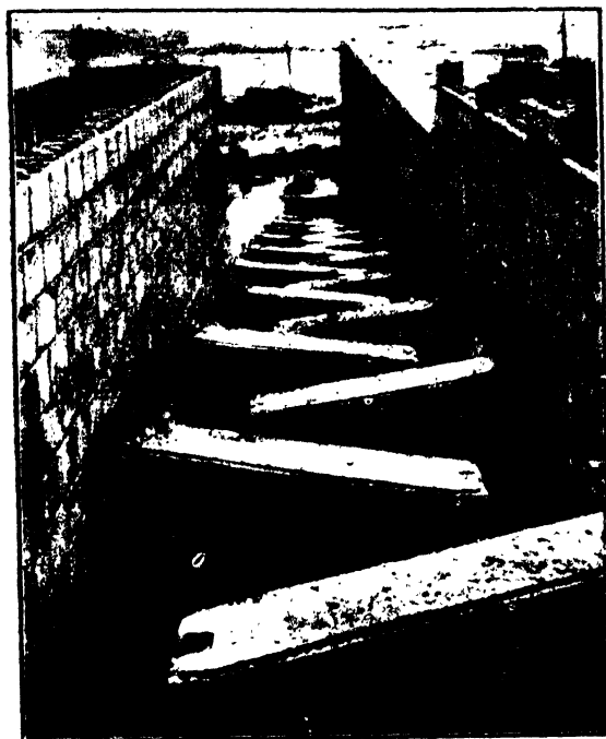
Fish ladder along Trimmu Weir Wall under construction. Fig. 10 (a)
