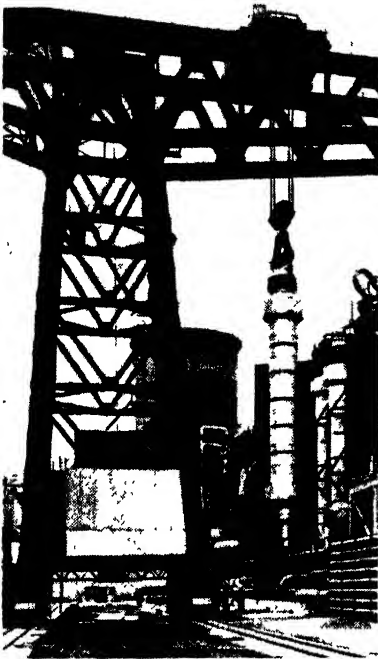
Figure 69.—Lifting a 160-ton converter in the I.C.I. hydrogenation plant
