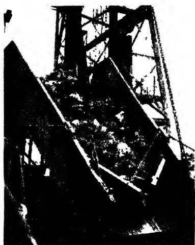
Figure 30.—Coal chute anti-breaking
