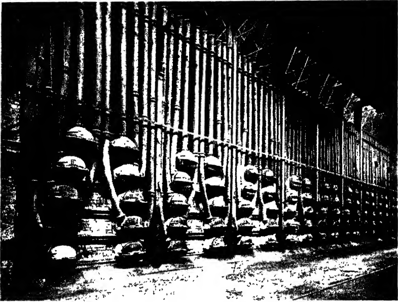
Figure 57.—Battery of horizontal gas retorts showing metal doors and gas off-takes
