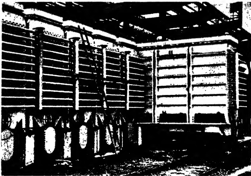
Figure 71.—FISCHER-TROPSCH PLANT IN GERMANY. Atmospheric-pressure reaction vessels during installation
