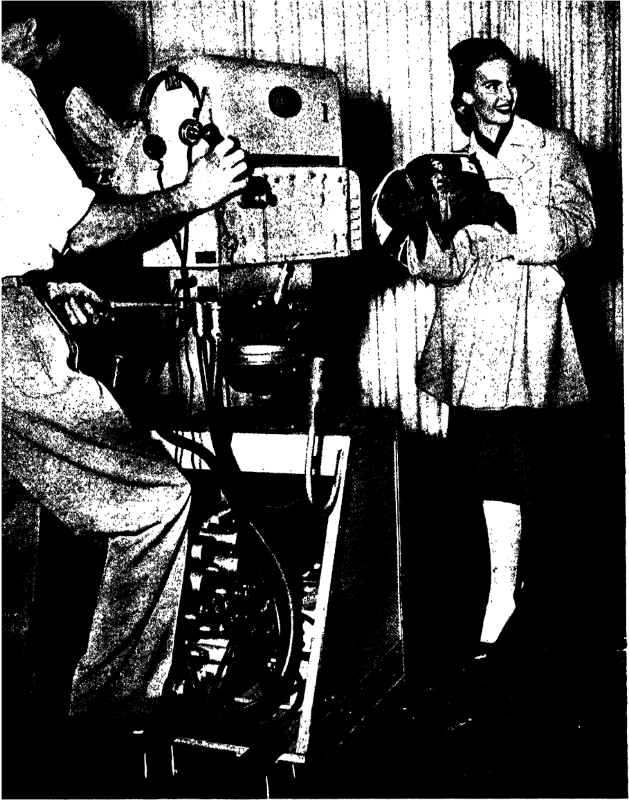
PLATE XVI.—An example of a relatively immobile floor-bound studio camera used at Du Mont during the war. Note awkward mounting on four casters, bulk of wires, tubes, and box. Note also view finder into which cameraman is peering. This is an electronic view finder which is a small television screen tapping the camera amplifier. Focusing on this camera is accomplished by pushing lever ( at right ) forward and backward. Routine of studio operations is marked on paper clipped to back of camera. Camera head itself is mounted on a motion-picture type of device which emits whirring noise when panned. This camera is limited to pans and tilts through a limited range. Raising the camera or dollying while the program is on the air is not practical.
