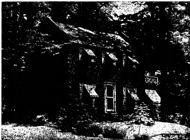
FIG. 42.—House at Dobbs Ferry, N. Y., with all-Rolok walls, Flemish bond. (Courtesy of Theodore Meyer, Architect.)
