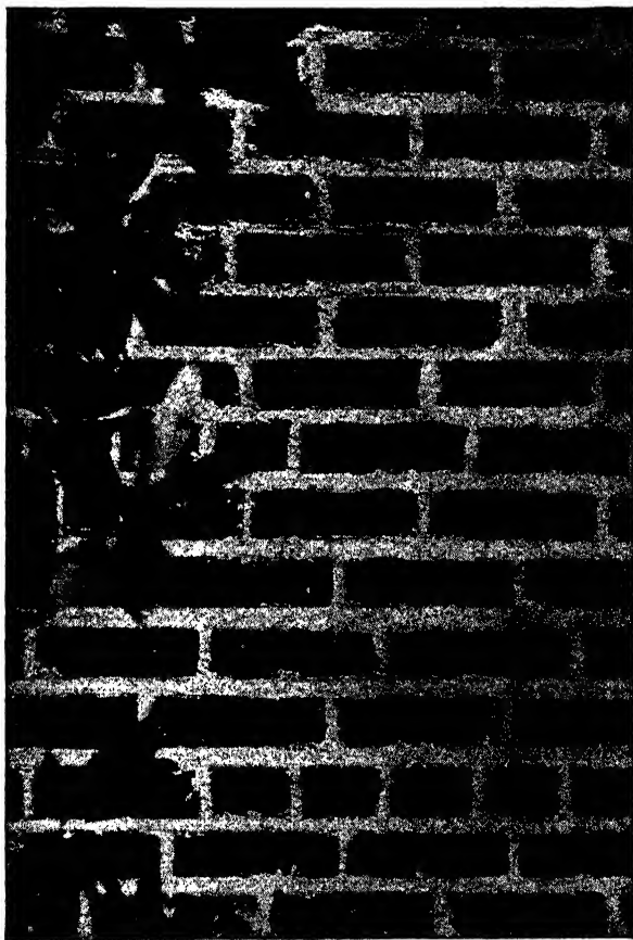
FIG. 40.—The Rolok-Bak wall does not reveal its construction on the exterior, its surface appearance being identical with that of the solid wall.
