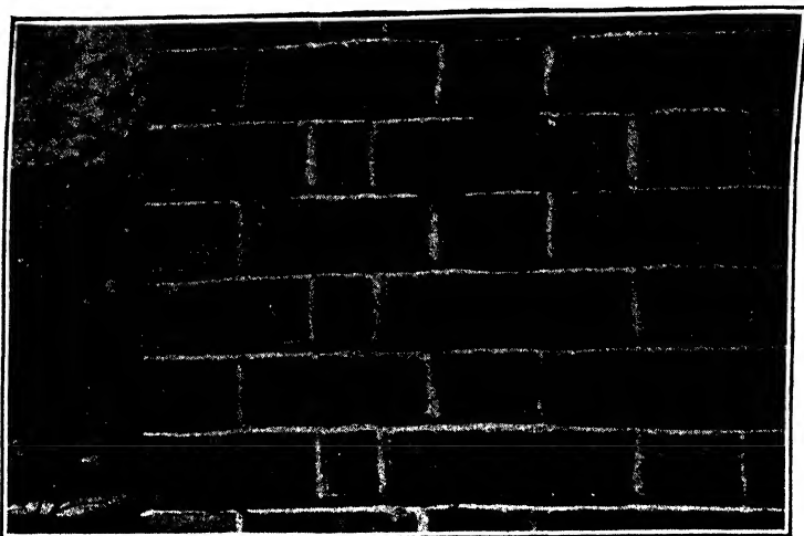
FIG. 20.—Concave joint in Flemish bond.
