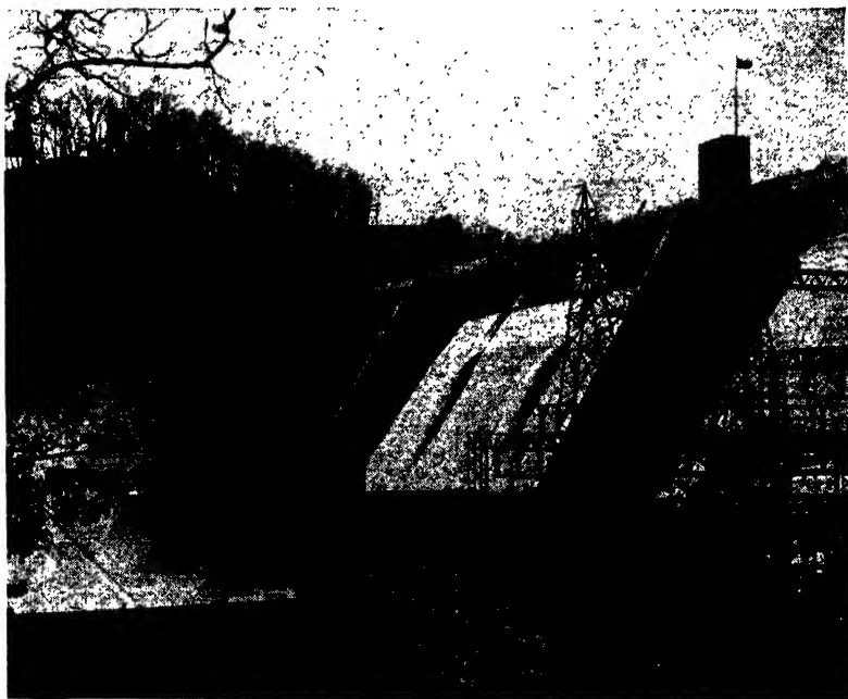
FIG. 13.—Norris Dam of the Tennessee Valley Authority. Dam is 265 ft. high, 1,860 ft. long. Reservoir area is 40,200 acres with useful storage of 2,020,000 acre-feet. Power house is of conventional type. ( Tennessee Valley Authority. )
