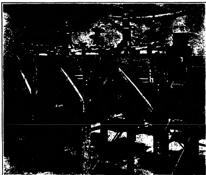
FIG. 215.—Outdoor oil circuit breaker, 70 kv., of the horizontal multibreak type. ( Pacific Electric Manufacturing Company. )
