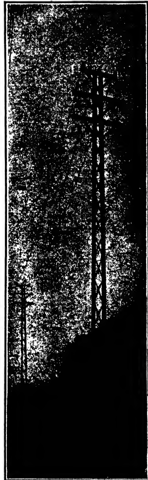
FIG. 273.—Steel-poleline. (Truscon Steel Company.)
