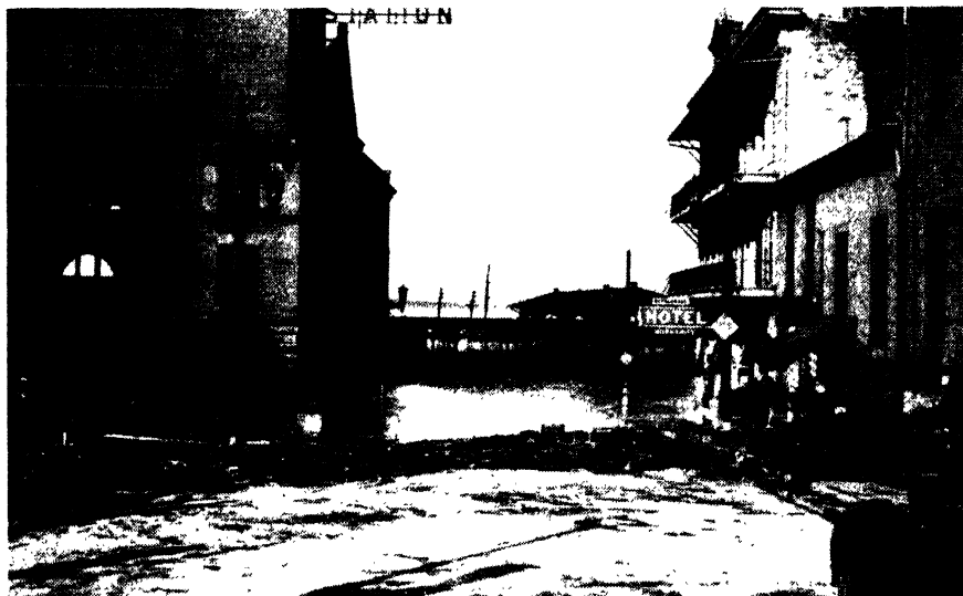
FIG. 7-4. Flood of February, 1937, Ohio River at Louisville, Ky.
