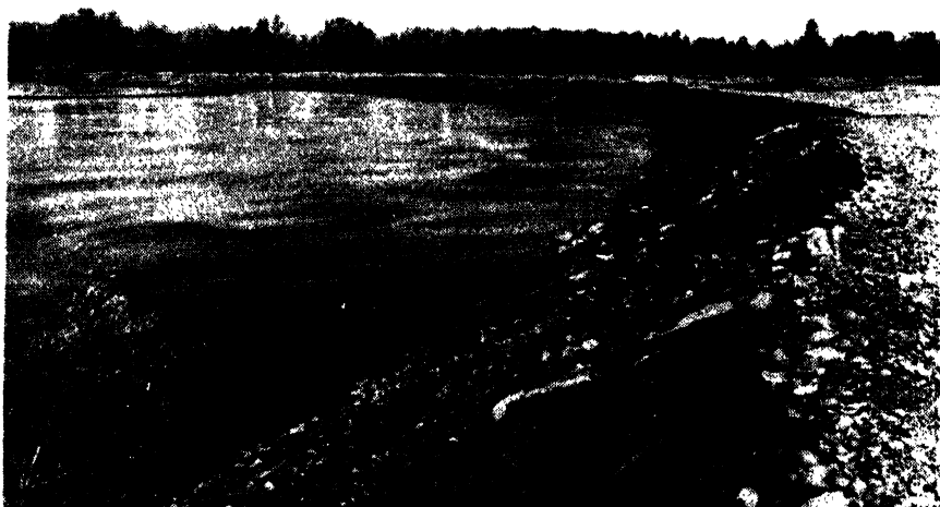
FIG. 15-3. Bank protection, Long Tom River.
