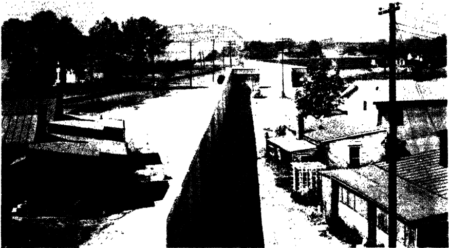
FIG. 18-16. Flood wall and closure section, Jeffersonville-Clarksville project.
