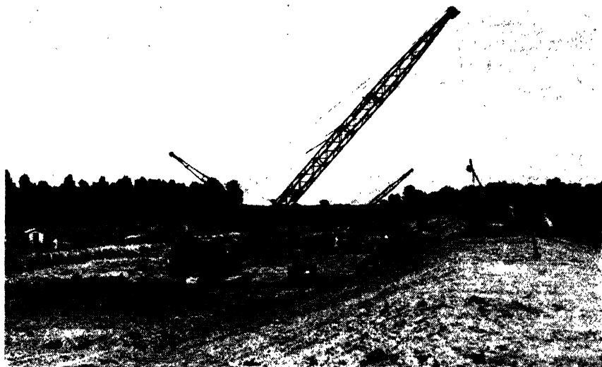
FIG. 10-13. Mississippi River. Levee construction.
