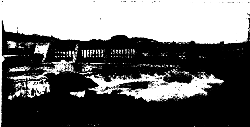
FIG. 6-5. Tainter gates and stanchion flashboards, Clarks Falls Dam.
