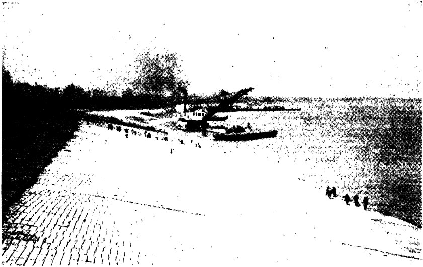
FIG. 10-9. Mississippi River. Concrete revetment at Milliken Bend.
