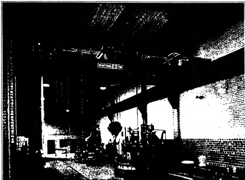
Fig. 151. Crane Girder Runways Supported on Brackets Courtesy of Whiting Corporation, Harvey, Illinois
