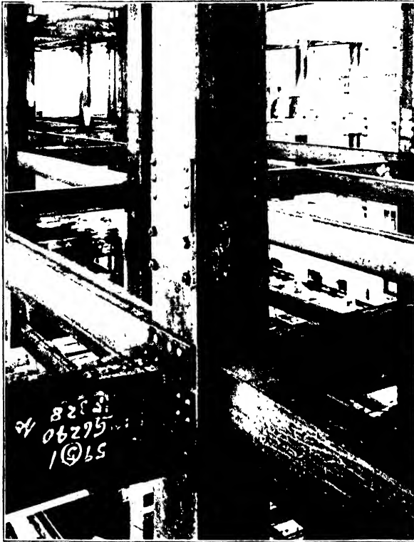
Fig. 216. Wind-bracing on an Interior Column Courtesy of The American Bridge Company
