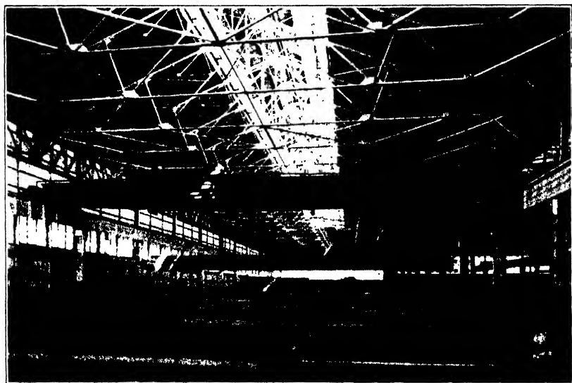
Fig. 139. Typical Mill Building with Fink Roof Trusses and Crane Courtesy of Whiting Corporation, Harney, Illinois
