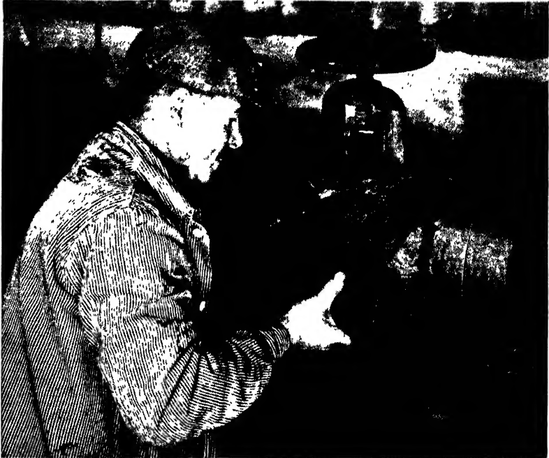
FIG. 96.—Method of insulating valves and fittings with rock wool. (Courtesy of the Johns-Manville Co.)
