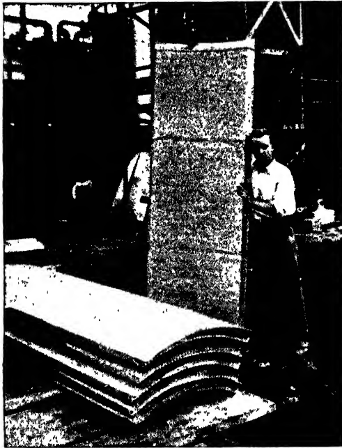
FIG. 111.—All-metal aluminum-foil panels. (Courtesy of the Alfol Insulation Co.)
