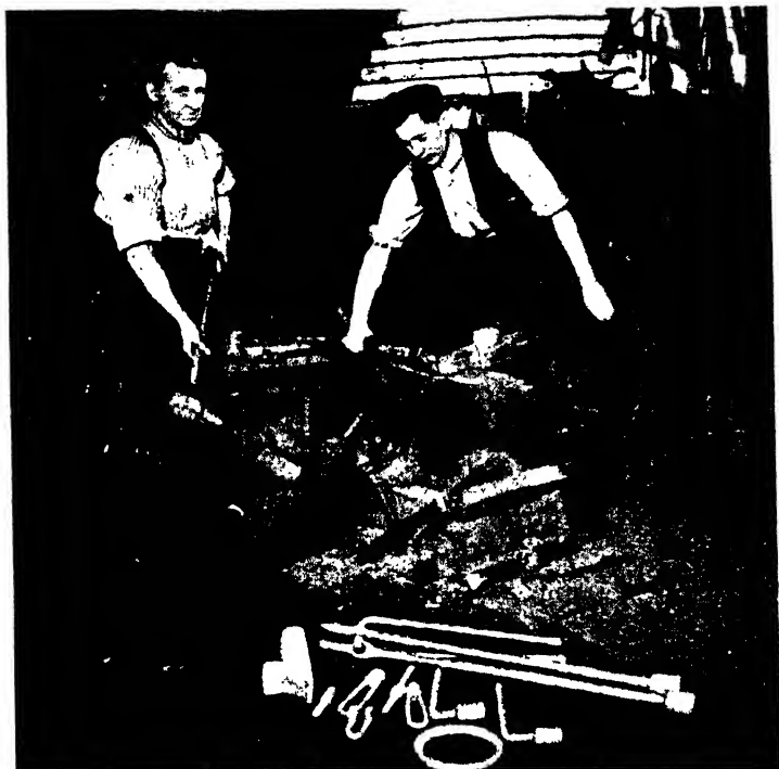
FIG. 179. APPRENTICE SMITH USING A TOP SWAGE, ASSISTED BY AN ADULT STRIKER
