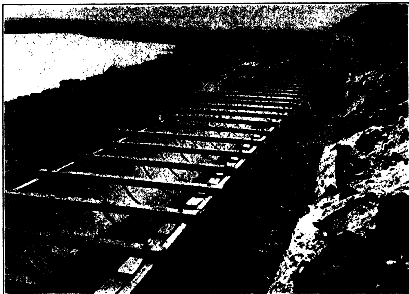
FIG. C.—Hess steel flume—7 feet diameter. Mountain Home Cooperative Irrigation Co., Idaho.
