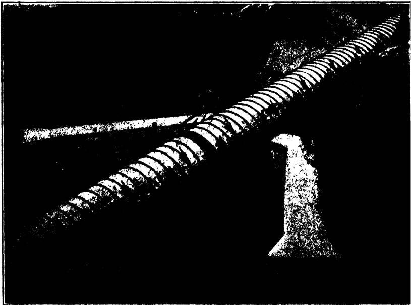
FIG. D.—Anchor on 42-inch pipe line. Tacoma, Wash. (Washington Pipe & Foundry Co.)
