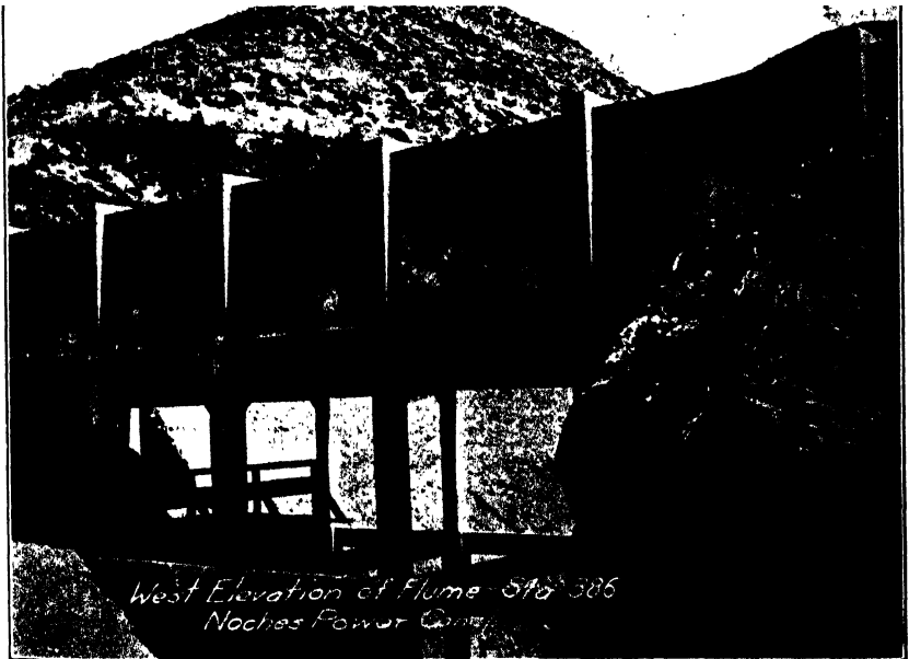
FIG. B.—Reinforced concrete flume. Naches Power Canal, Wash.
