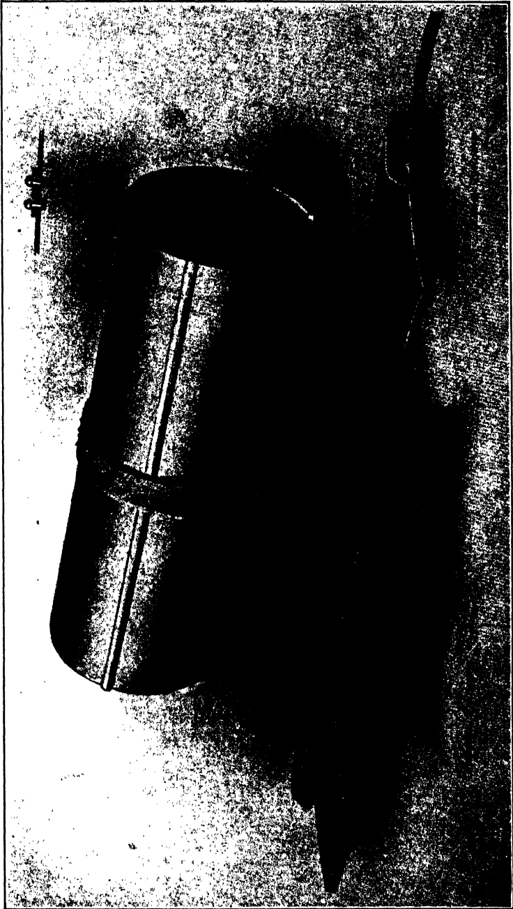
Fig. A.—Details of lock-bar steel pipe.
