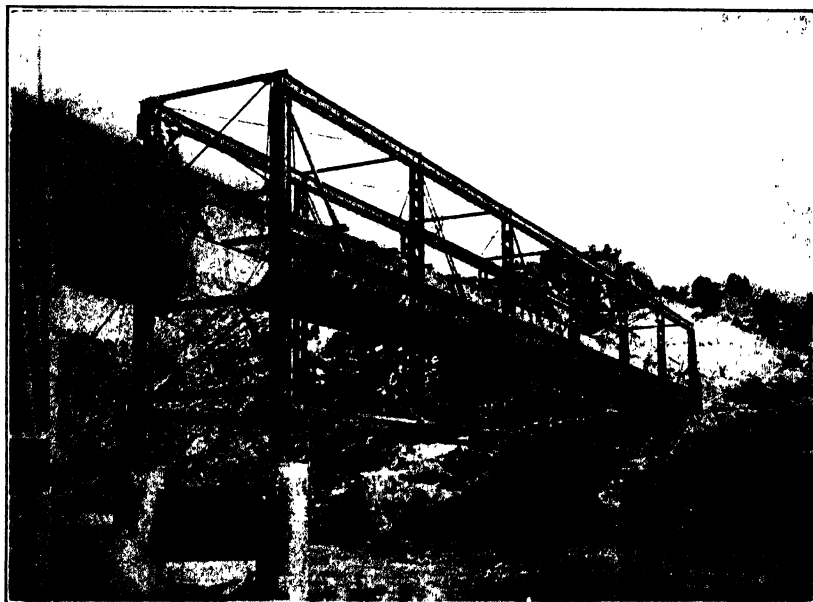
FIG. D.—Lennon steel flume, 9 feet diameter on 110-foot span steel bridge over Las Animas River, Cedar Hill, N. Mex., for Aztec Irrigation Co.
