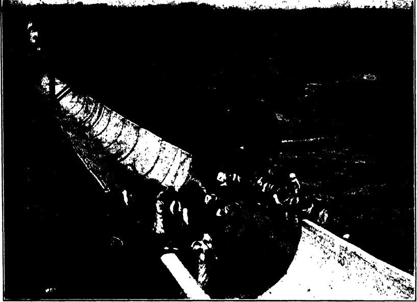
FIG. A.—Placing steel tubes surrounded with outside reinforcement, in cradles. Sosa Siphon, Spain.
