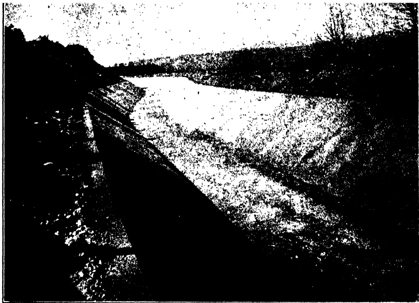
FIG. C.—Concrete-lined canal. Ridenbaugh Canal, Idaho.
