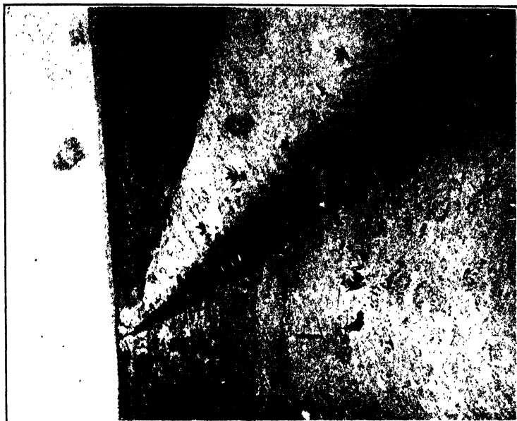
FIG. B.—24-inch machine banded wooden stave pipe. Eastern Washington (Washington Pipe & Foundry Co.).
