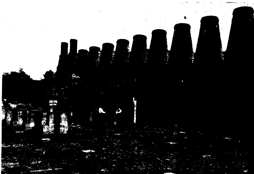
Figure 2. A battery of abandoned vertical cement kilns of the Giant Portland Cement Company, at Egypt, Pennsylvania.
