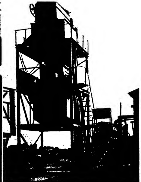
FIG. V.14. —Bitumastic Macadam Plant, showing Dryer (in background), elevator to screen and bins above, mixing platform, and storage bins for coated material.
