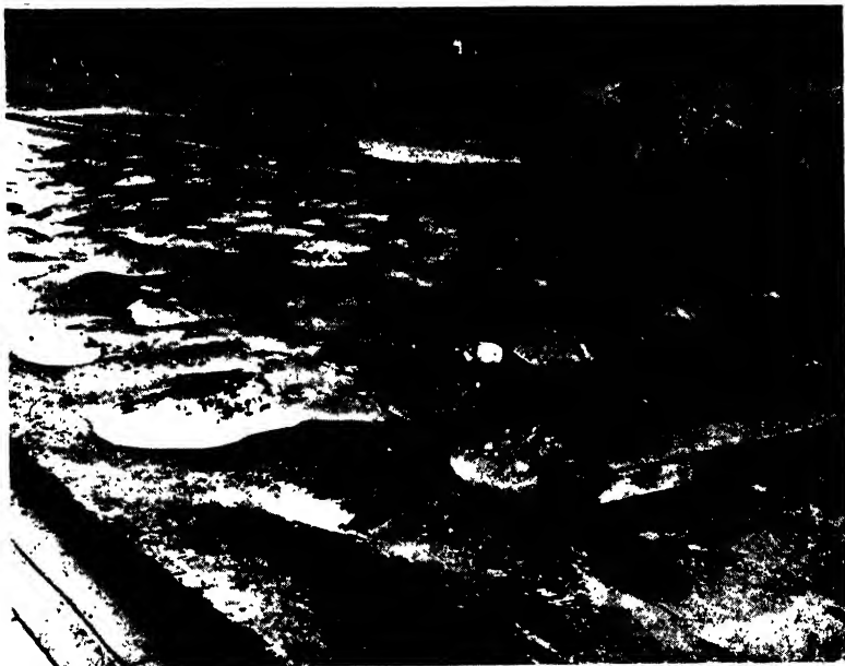
FIG. IX.1.—Result of a Burst Water Main under an Asphalt Surfaced Roadway.
