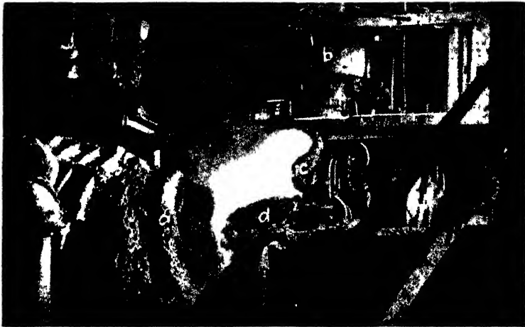
FIG. VI-9.—Pouring metal into the converter. (a) Converter, (b) cupola, (c) ladle, (d) runner
