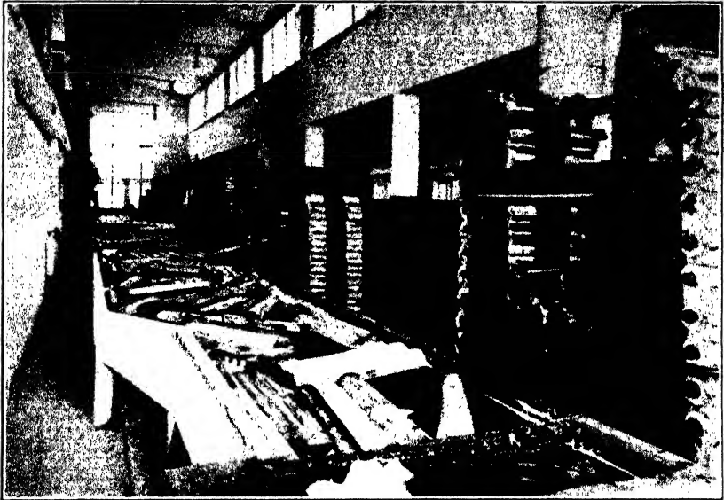
FIG. 34. CHARGING FLOOR. CONTINUOUS-CHAIN-GRINDER INSTALLATION. Finland.
