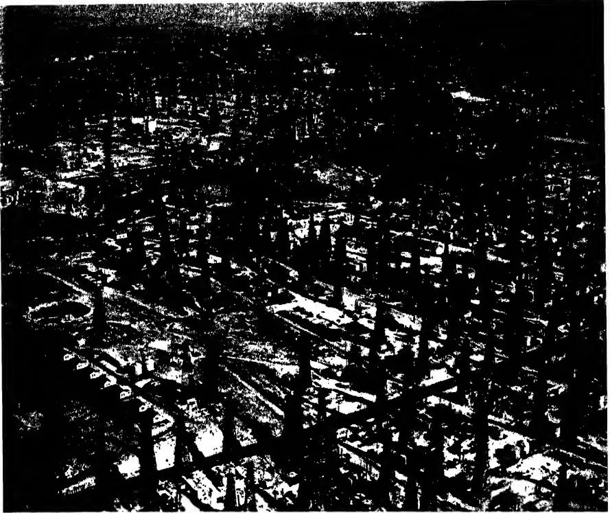
286. Signal Hill oil field, near Los Angeles, Calif. This is one of the highly productive California oil fields, developed in Tertiary rocks. The anticlinal structure that controls accumulation of the oil is topographically expressed by the broad hill. ( Spence Air Photos. )
