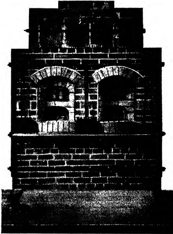
FIG. 6. Twin double-muffle soft-coal furnace.
