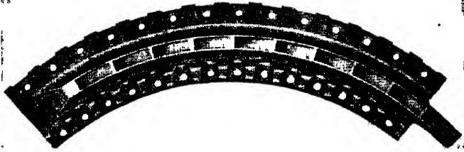
FIG. 148. First-stage nozzle plate for a Curtis turbine
