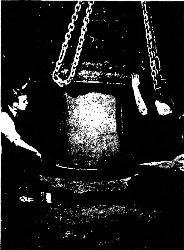
FIG. 17B. ASSEMBLING THE CORE IN THE MOULD (Council of Ironfoundry Associations)
