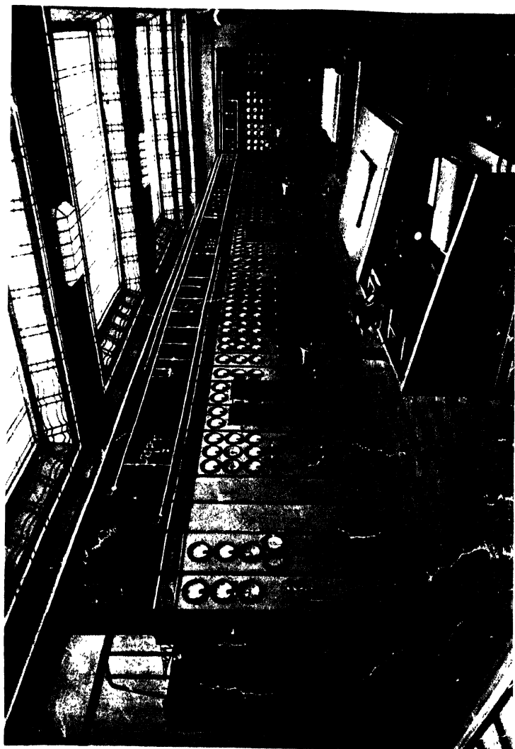
• PART OF THE CONTROL ROOM OF A BRITISH POWER STATION.
