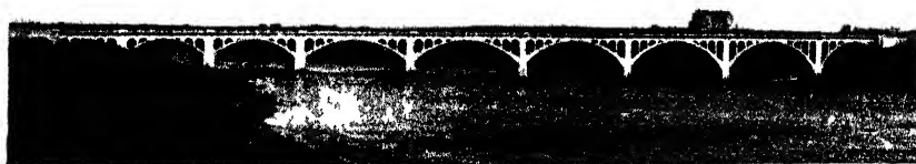
Fig 373 – Bridge in Saskatoon, Canada
