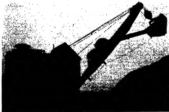
Fig. 280. —Excavating with a Mechanical Shovel.
