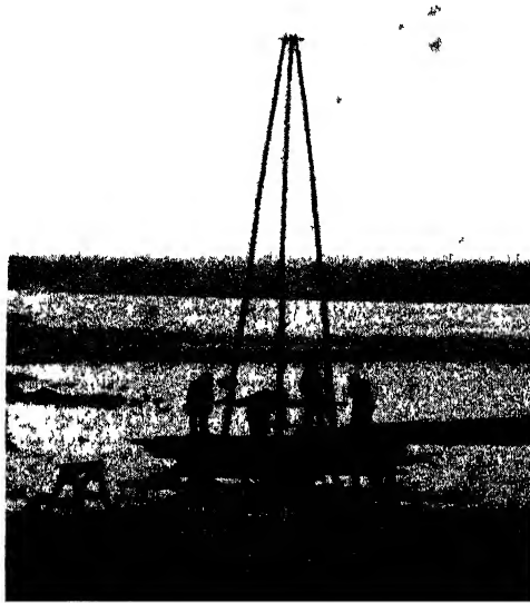
Fig. 14.—Winch Boring in Progress.
