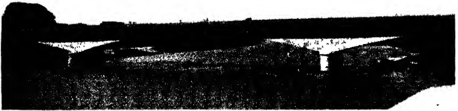
Fig. 365.—Bridge at Villeneuve-St. Georges, France.
