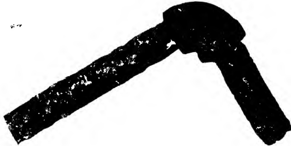
Severe Corrosion Apparently the Effect of Dissimilar Metals with Probably Some Electrolysis
