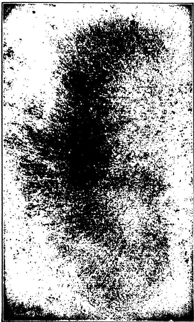
FIG. 344A.—About right amount of asphalt.
