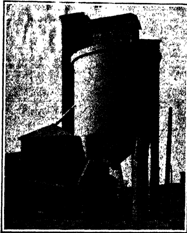
FIG. 186.—A reinforced concrete sand bin.
