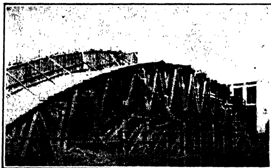
FIG. 209.—Pile bents used as centering.
