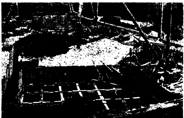
FIG. 244.—Telescoped sheet piling coffer-dam.
