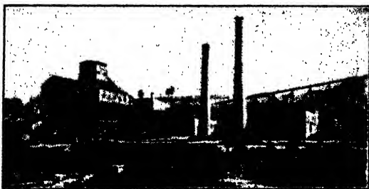
FIG. 12.—Shaft house and tipples, bituminous coal mine, Spring Valley, Ill.
