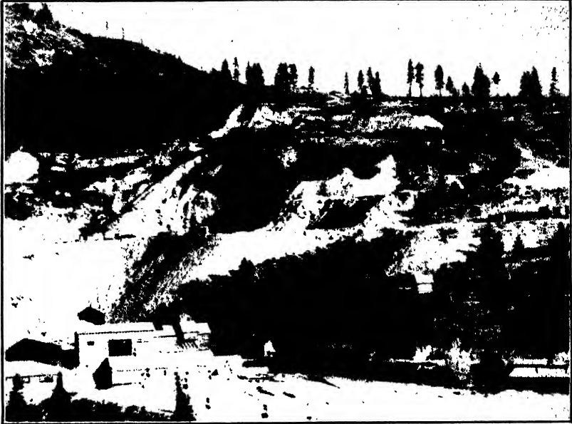
FIG. 1— Finch magnesite quarry near Chewelah, Wash. (Courtesy Northwest Magnesite Company.)
