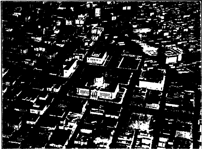
FIG. 126.—Air view of the civic center of San Francisco.
