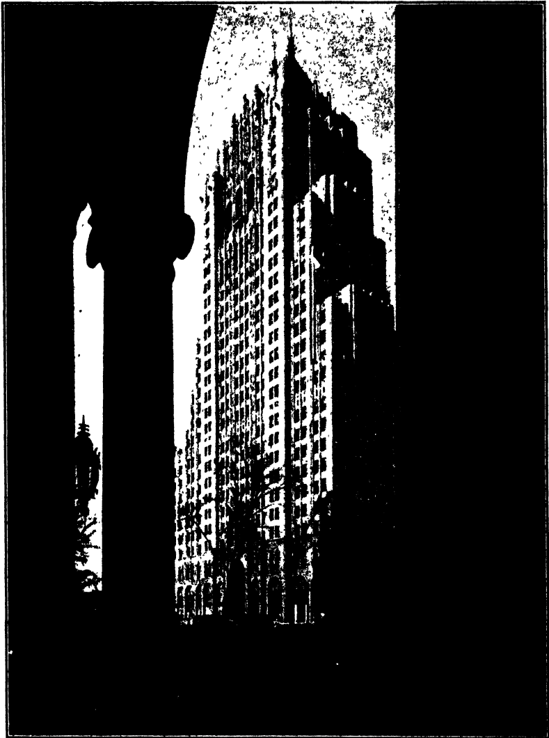
FIG. 120.—The Fisher Building, Detroit. The most outstanding contribution to Detroit's fast-growing skyline is the Fisher Building. It rises to 440 feet and is constructed almost entirely of granite and marble. (Courtesy of Fisher Building Corporation, Herbert A. Fisher, Manager.)
