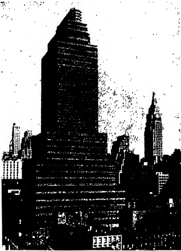
FIG. 47.—Hood, Godley, and Foulhoux. The McGraw-Hill building (completed 1931). Steel frame construction, 33 stories and basement. New York.
