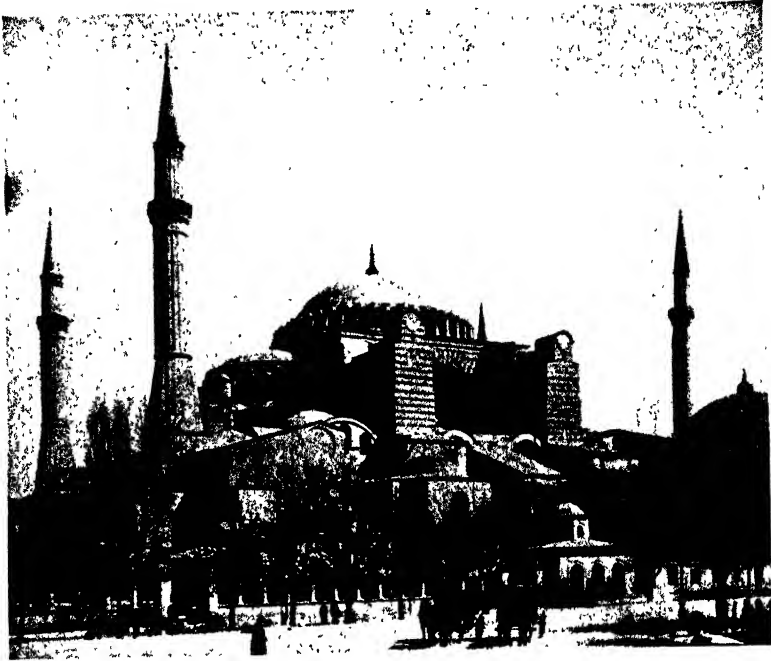
FIG. 149.—Anthemius of Tralles and Isidorus of Miletus. Santa Sophia (532-537) (restored 558, 975). Minarets added in fifteenth and sixteenth centuries. Brick and cement. Length: 247 feet; width: 231 feet; height: 184 feet. Constantinople. (New York University.)
