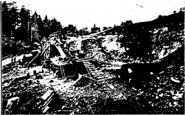
FIG. 2-2.—A roadside stone quarry with temporary crushing and screening plant.
