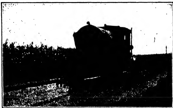
FIG. 7-18.—Applying oil to earth road.
