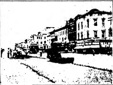
FIG. 13-2.—Resurfacing old brick with sheet asphalt.
