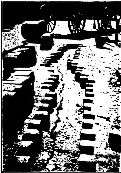
FIG. 9-27.—A crack in the base of a brick pavement. Mesh reinforcement would have prevented this crack from widening, the cushion from leaking, and the brick from settling. Repaired by cleaning out and filling with asphalt.
