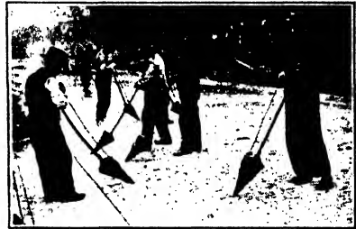
FIG. 10-8.—Applying asphalt filler with conical pouring can.
