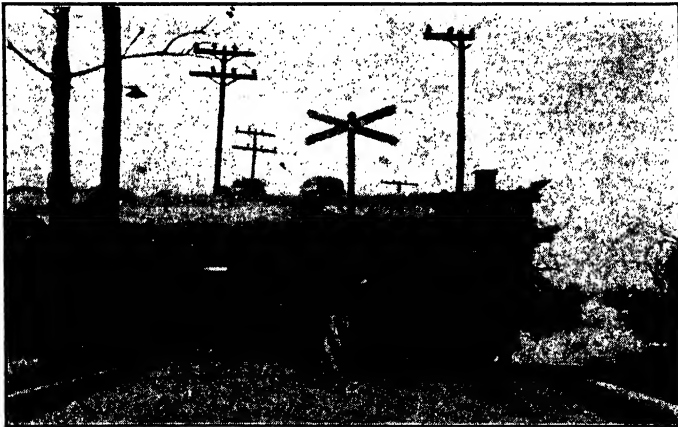
FIG. 20-6.—A good signal in the wrong place. Note the restricted traffic lanes and the obstruction the signal offers to movement in emergency.
