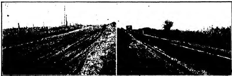
Before. After. FIG. 8-10.—Scarified, regraded, and dressed with ¾ in. of pea gravel.
