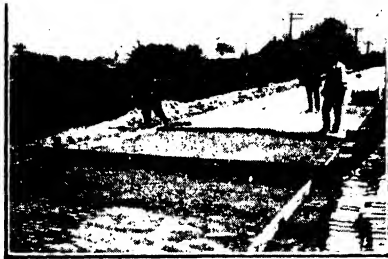
FIG. 13-3.—Adding new monolithic brick top to old brick road.
