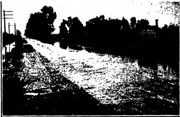
FIG. 5-2.—The result of inadequate outlet for the side ditches.
