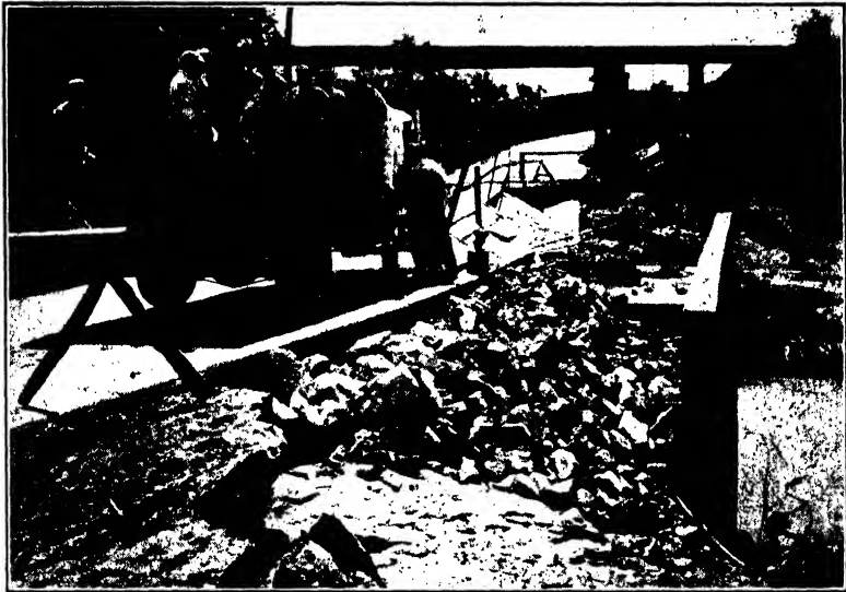
FIG. 13-11.—Washouts often demand repairs of many kinds.
