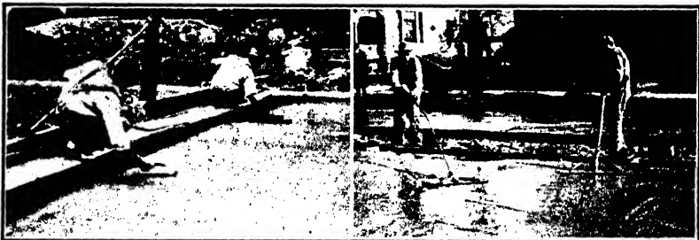
A B FIG. 9-3.—A, hand floats; B, long-handled floats.
