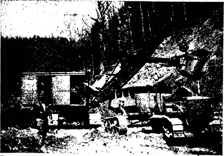
FIG. 6-9.—A gasoline power shovel loading a dump wagon pulled by a tractor. All three machines have caterpillar treads.
