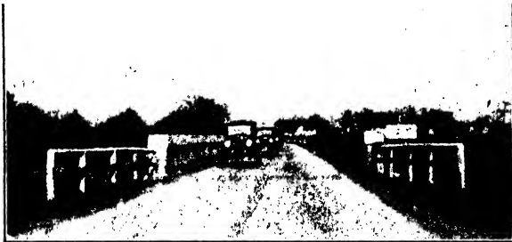
FIG. 16-13.—Evidence of the need for greater width of bridges. Traffic crowds to the center on account of the high girders. The oil streaks on the pavement are about 2 ft. closer together on the bridge than elsewhere.
