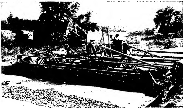
Fig. 9-4.—A finishing machine making the second run over the surface.
