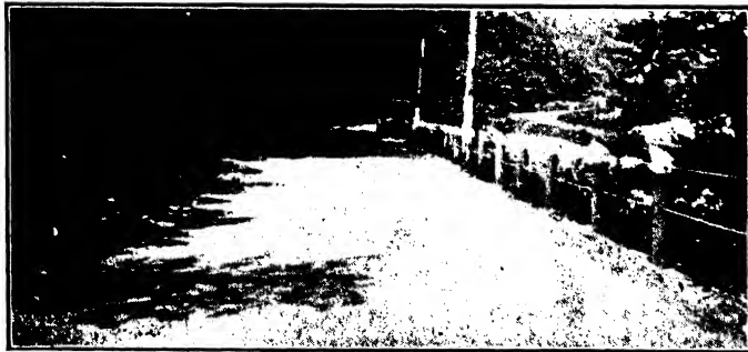
C. The road after a few days of use. FIG. 11-6.—Tar retread.
