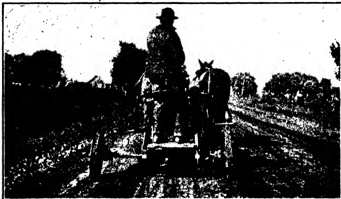
FIG. 7-11.—Patrol grader at work. Note the direction in which the dirt is being moved to preserve the correct crown.
