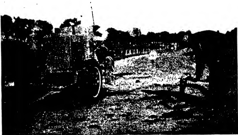
FIG. 9-22.—Poulter mudjack.
