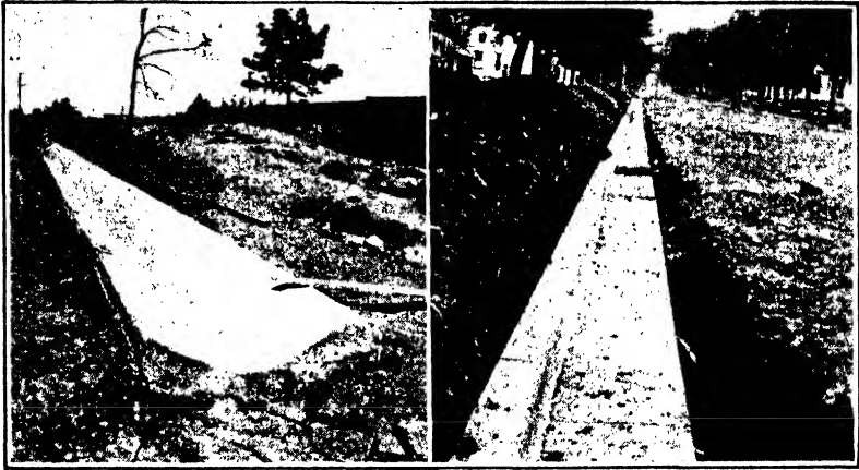
FIG. 12-1.—The deep V-gutter and the combined curb-and-gutter.
