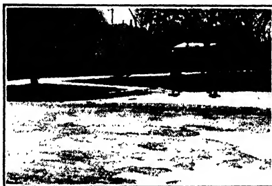
FIG. 9-12.—Surface scaling.
