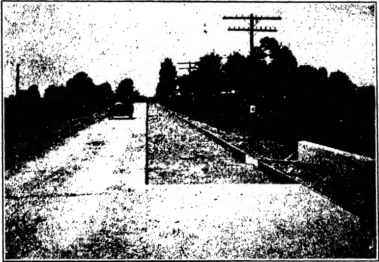
FIG. 16-4.—Double tracking an existing pavement.
