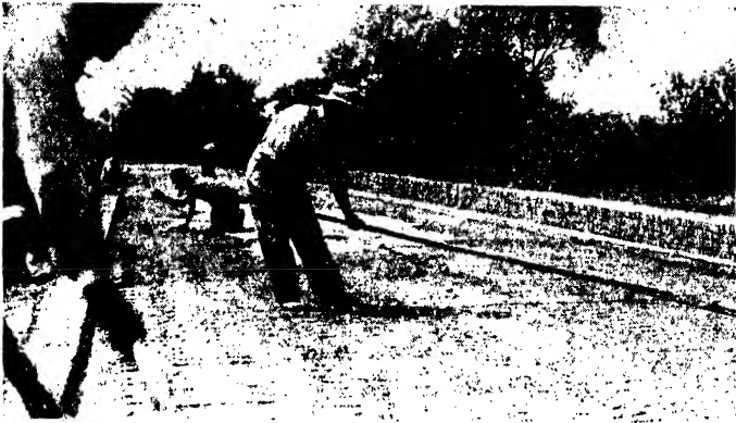
FIG. 13-5.—Truing a widened concrete slab with cement mortar preparatory to adding a brick surface.
