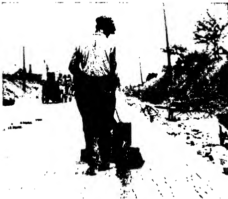
FIG. 10-9.—Applying asphalt filler with the squeegee buggy.
