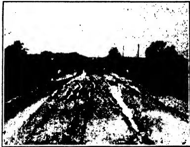
FIG. 7-12.—Mud hole near culvert caused by V-leveler.
