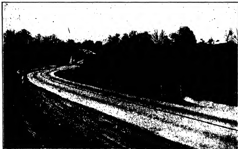
FIG. 14-8.—Modern alinement at subway to give good sight distance. Built in 1924. Note also the absence of a center support in the subway.
