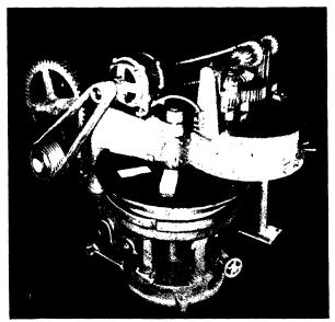
Fig. 87.—Looking down on Model "C" Jackson brick machine.
