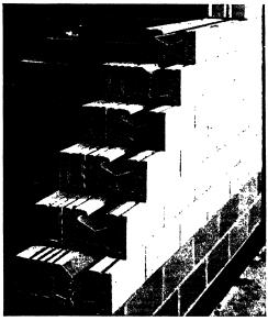
Fig. 138.—Natco Dri-speedwall Tile hollow masonry. For 12-in. wall construction.
