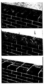
Fig. 41.—Methods of bonding. Top, metal ties; center, diagonal headers; bottom, bonding brick (8 by 8 in.).
