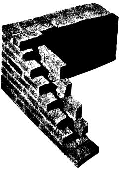
Fig. 134.—Eight-inch Rolok-Bak wall. Six courses of the outside 4-in, withe are first laid, backing up with the inside withe of brick on edge, and the continuous header course of brick laid flat is next placed.
