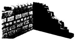
Fig. 135.—Eight-in. All-Rolok wall. Note the simplicity of this sturdy wall-two continuous courses of stretchers, front and back, followed by the header course.
