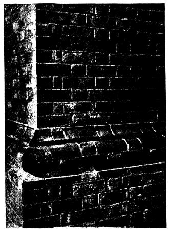
Fig. 93.—Special brick for *The Reader's Digest* Building near Chappaqua, N. Y. Architect, James C. Mackenzie.
