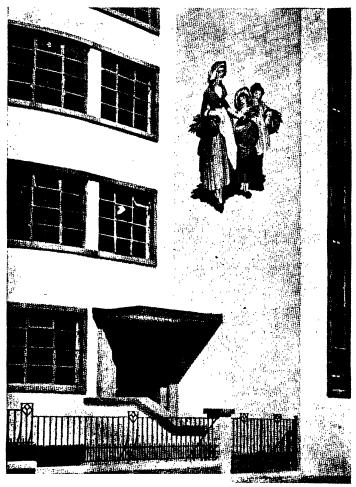
Fig. 139.—Faience and faience slabs on a factory building in East London, England. (R. Fitzmaurice, Principles of Modern Building, Vol. 1, Building Research Station, Garston, Herts.)
