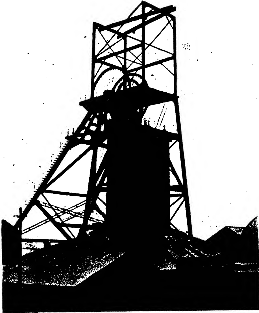
FIG. 64.—Steel Headgear of Rolled Sections.
