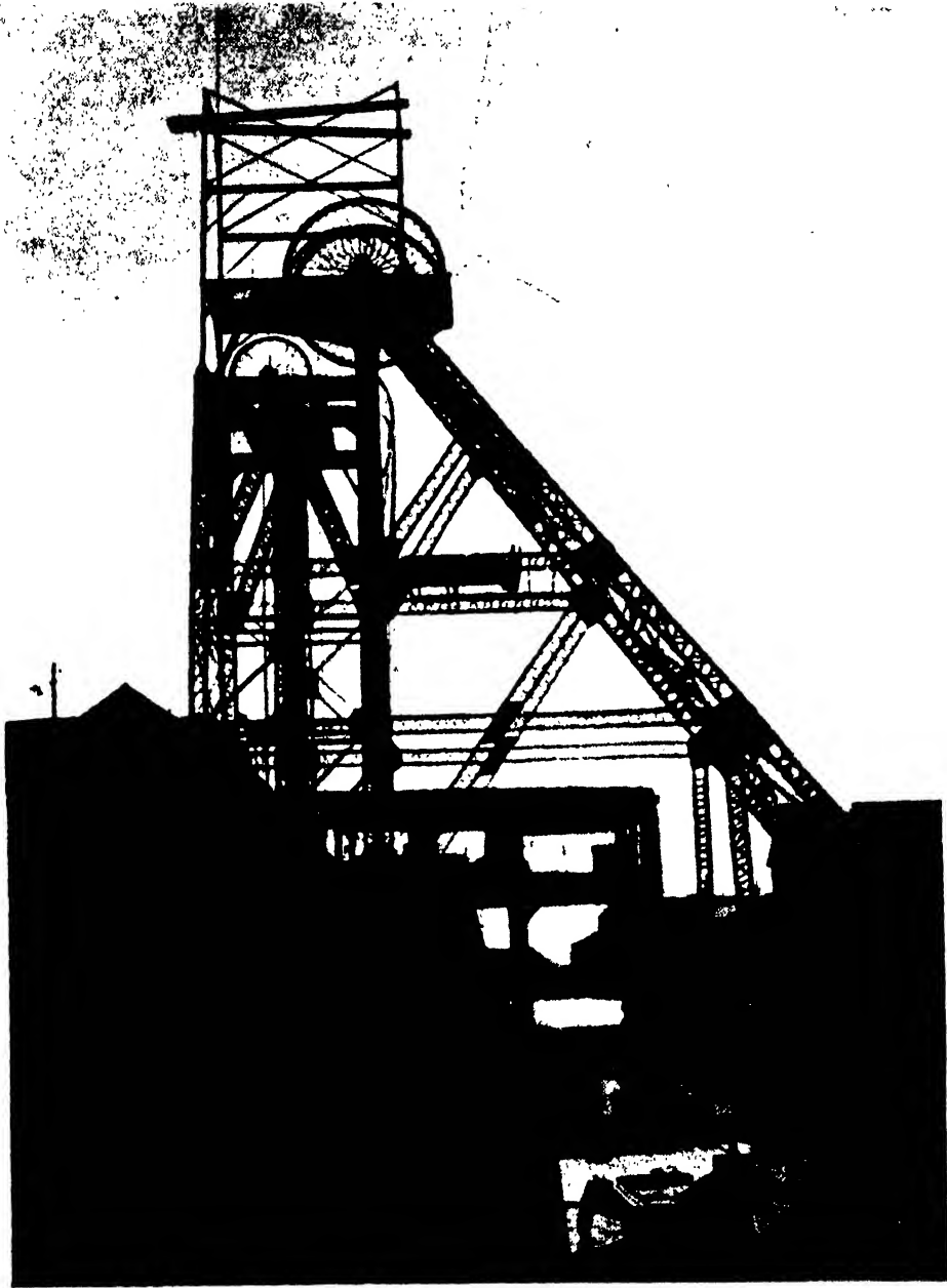
FIG. 63.—Steel Headgear of Lattice Girders.
