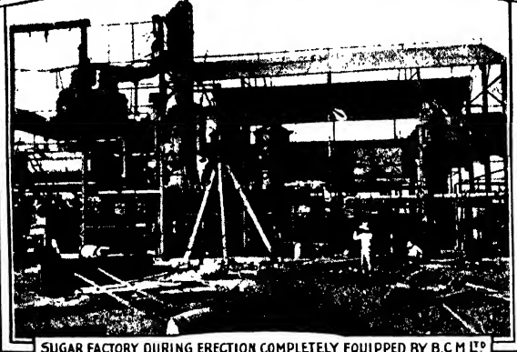
SUGAR FACTORY DURING ERECTION COMPLETELY EQUIPPED BY B.C.M. LTD.
