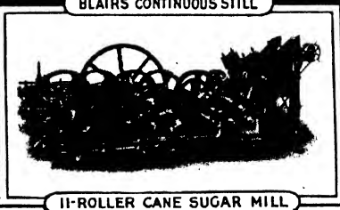
11-ROLLER CANE SUGAR MILL
