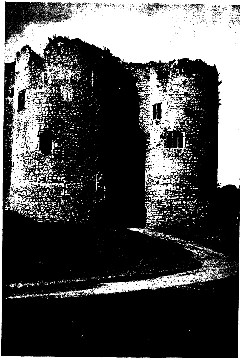
78 CHEPSTOW, MONMOUTHSHIRE: an early 13th-Century Gatehouse
