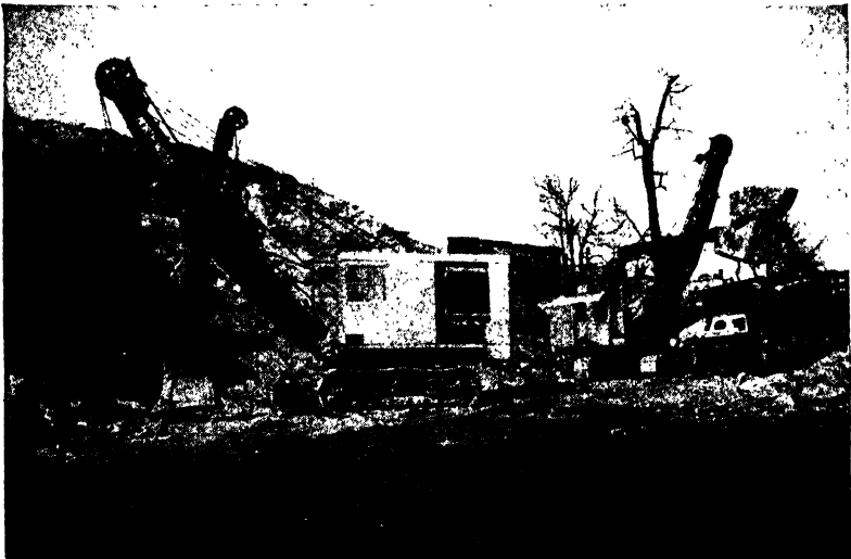
FIG. 7.—Northwest shovels in heavy rock cut for approach to George Washington Bridge, New York City. (Courtesy of Northwest Engineering Company.)
