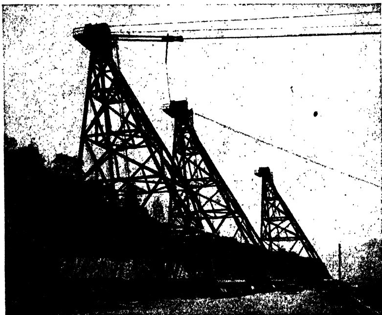
FIG. 20.—Tail towers for cableway at Shasta Dam. (Courtesy of U.S. Department of the Interior.)
