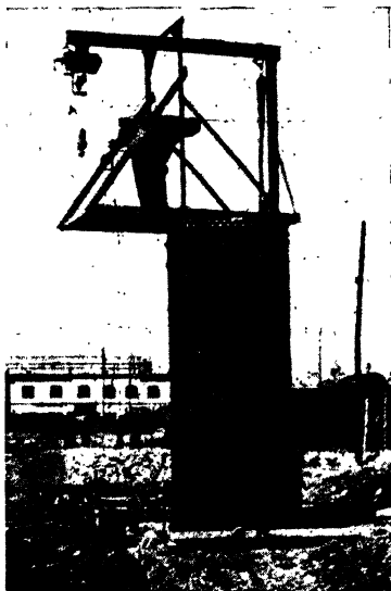
FIG. 19.—Open steel-cylinder caisson.
