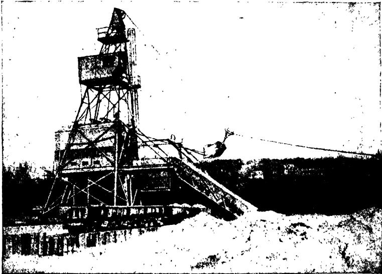
FIG. 15 b .—Dragline scraper with self-propelled head tower. (Courtesy of Saucerman Bros.)
