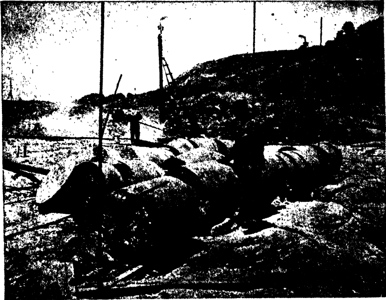
FIG. 12b.—Thirty-six-inch calyx cores. (Courtesy of Ingersoll-Rand Company.)
