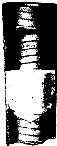
FIG. 40B.—Raymond standard-taper piles.
