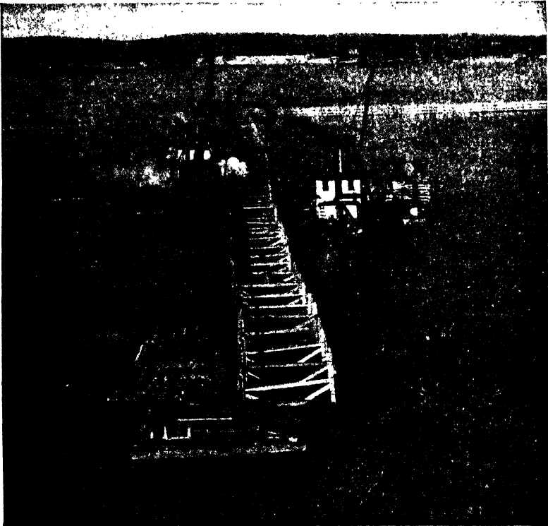
FIG. 6.—Ohio River type cofferdam at Wheeler Dam.
