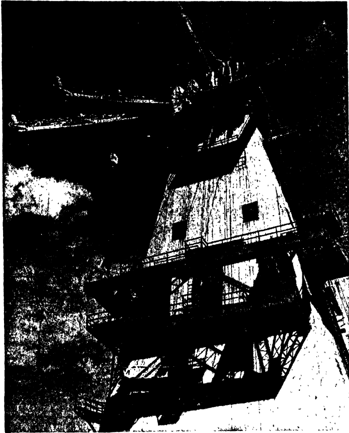
FIG. 21.—Head towers for cableway at Shasta Dam. (Courtesy of U.S. Department of the Interior.)
