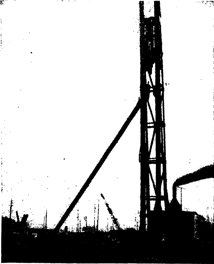
FIG. 43.—Sixty-foot monotube pile being placed in leads.
