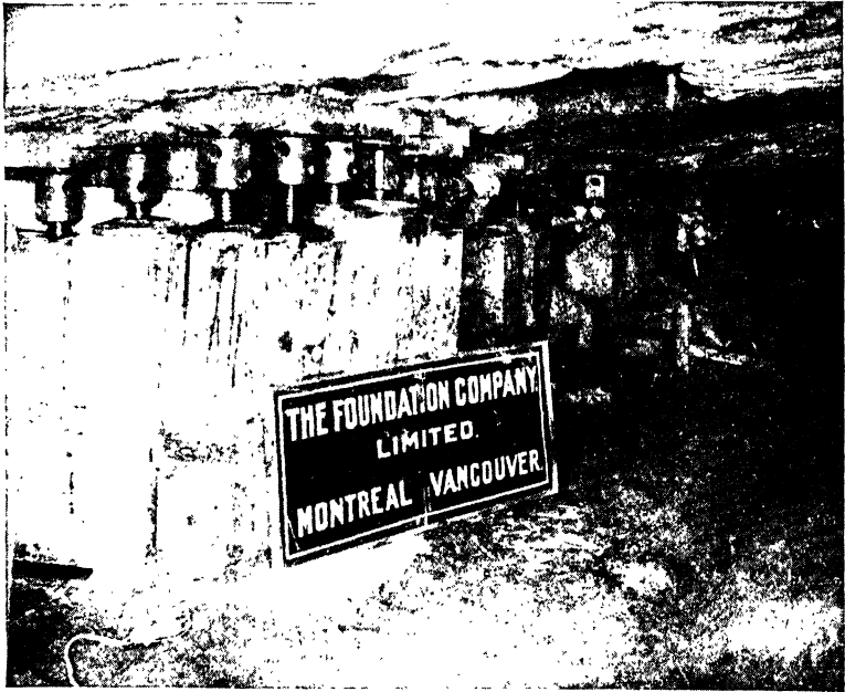
FIG. 20.—Jacking operations, Winnipeg grain elevator. (Courtesy of Foundation Company.)
