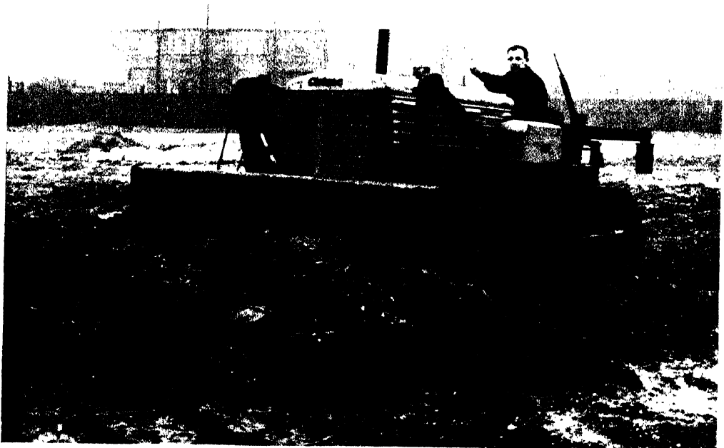
PLATE 3. 'Cletrac' Crawler Tractor and Bull-dozer engaged on levelling
