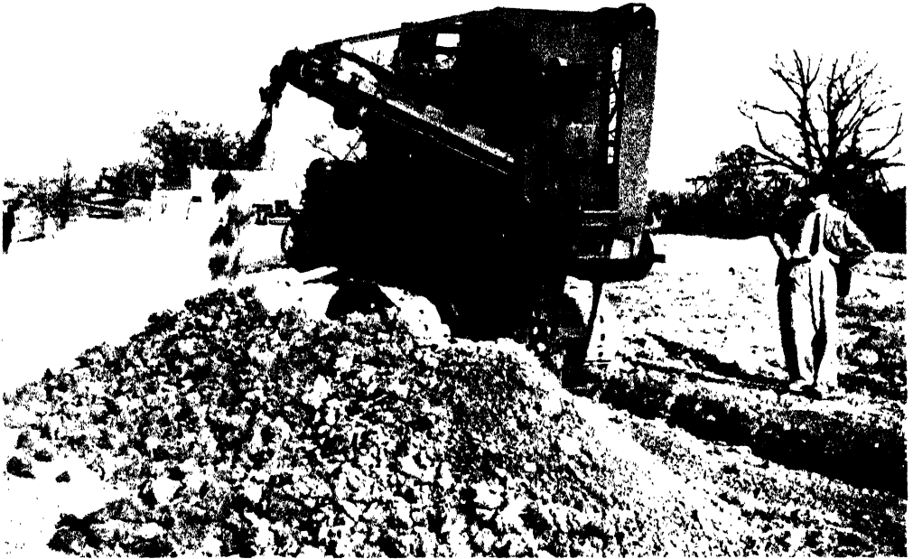
PLATE 12. A 'Barber-Greene' Ditcher at work excavating trench for land drains
