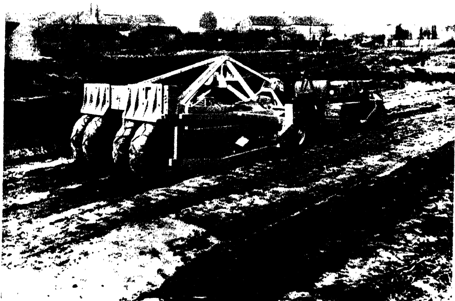
PLATE 5. Excavating by heavy Crawler Tractor and Scraper
