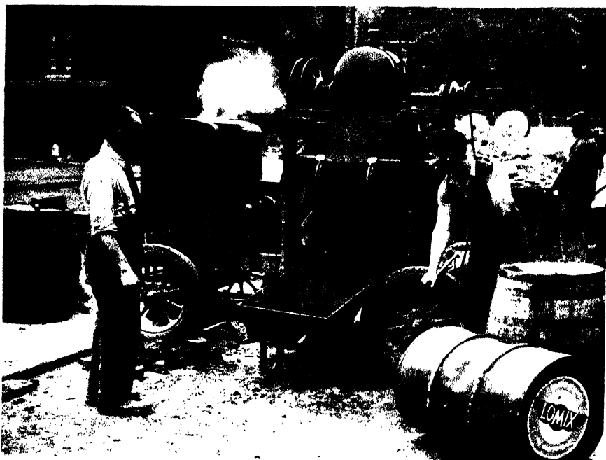
PLATE 28. Stabilized soil surface. Gauging and mixing materials
