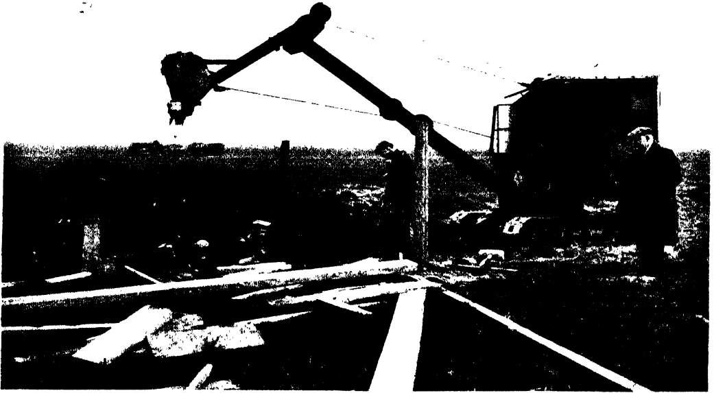
PLATE 14. A Back-Acting Excavator on trenching work
