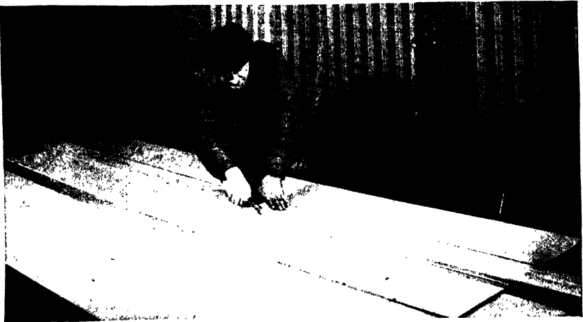
Fig. 11. Workman Scoring Sheetrock Board for Cutting or Breaking Courtesy of United States Gypsum Company, Chicago, Ill.
