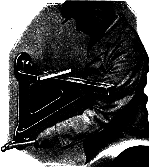
Fig. 19B (Right).—LEVELLING A WALL BRACKET Second operation.
