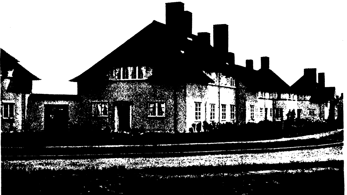
Two Similar Corner Treatments. THOMPSON, HENNEL and JAMES, Architects.
