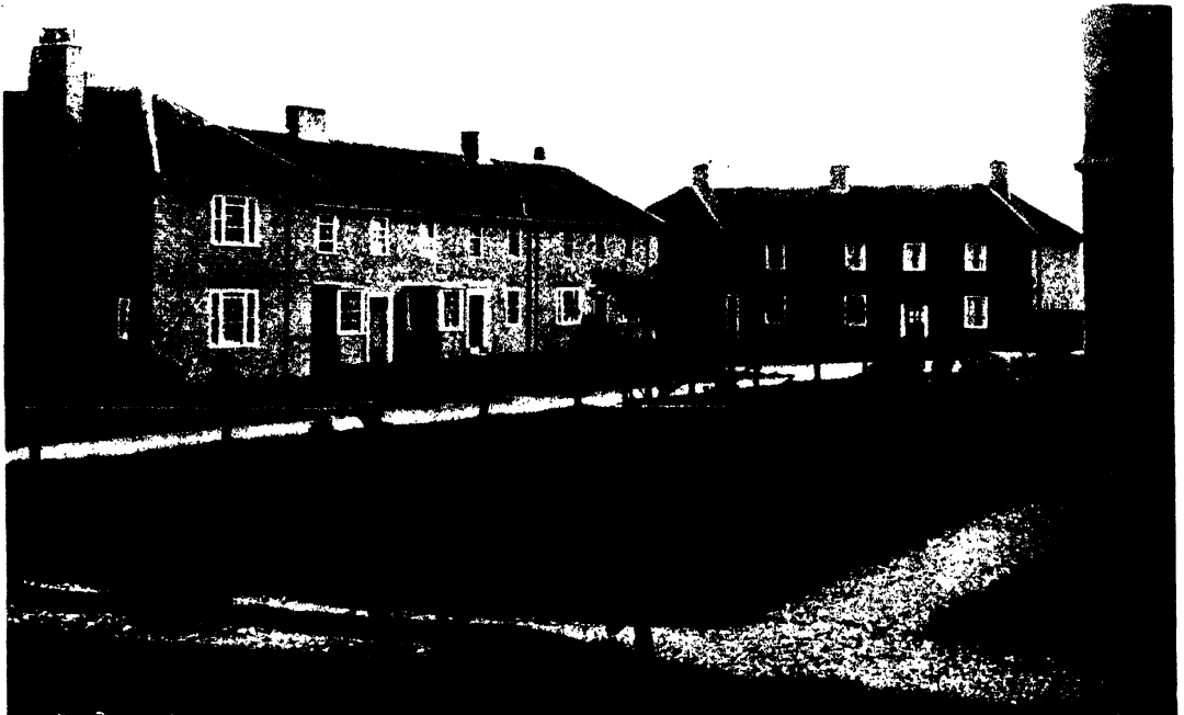
Two Views of Dellcot Close. The absence of front fences is to be noted.
