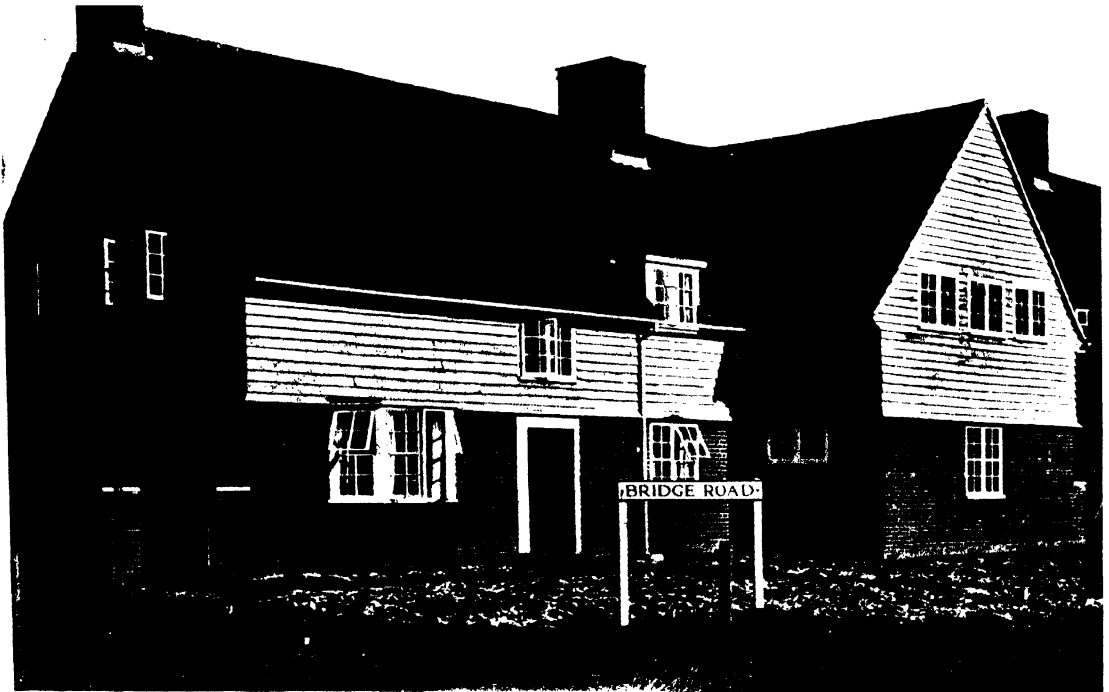
Elm weather boarding with bricks made on the estate. HENNELL and JAMES, Architects.
