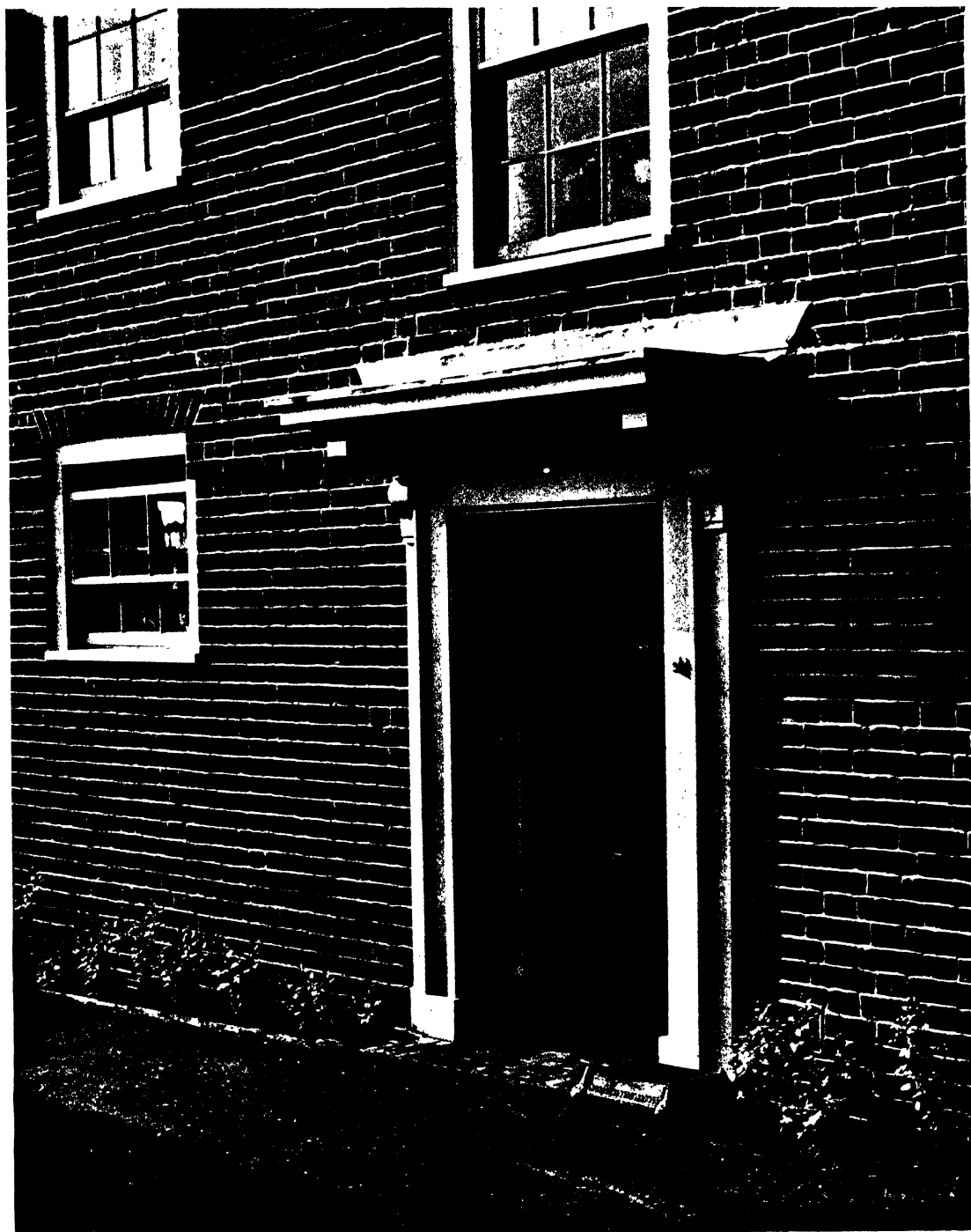
Detail of a Doorway.
