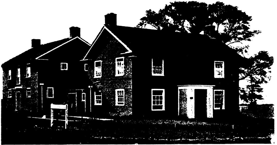
Two Detached Cottages linked by Outbuildings.
