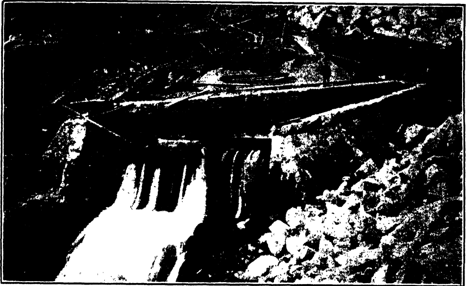
FIG. 102.—Rectangular weir with end contractions. (From a photograph by F. H. Fowler.)
