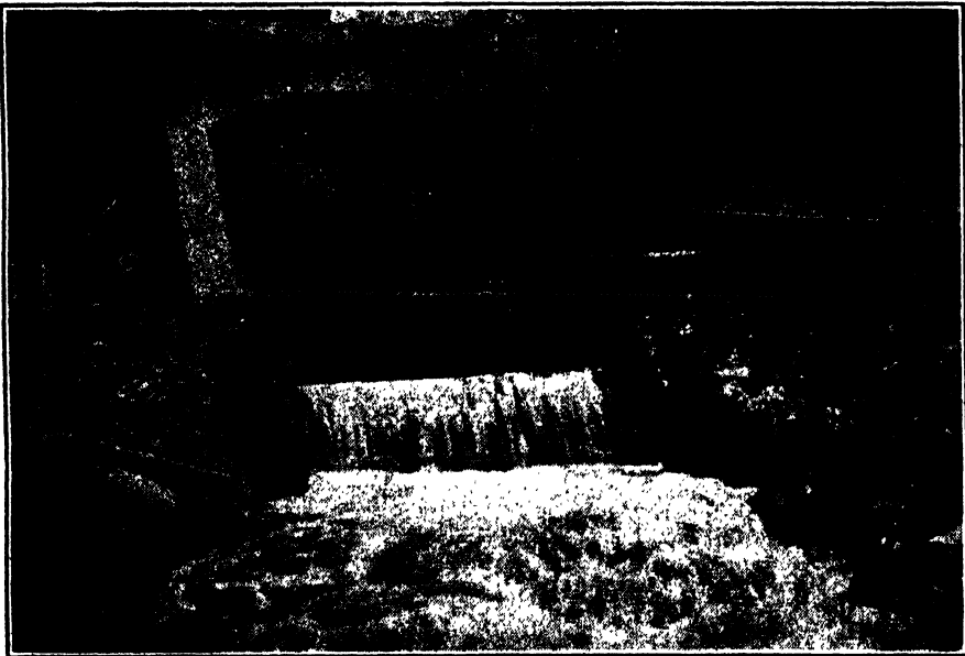
FIG. 101.—Rectangular weir without end contractions.
