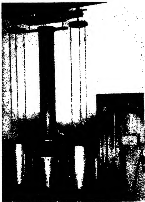
FIG. 7-3b. Torsion-balance arrangement for the determination of the gravitational constant (after Heyl).
