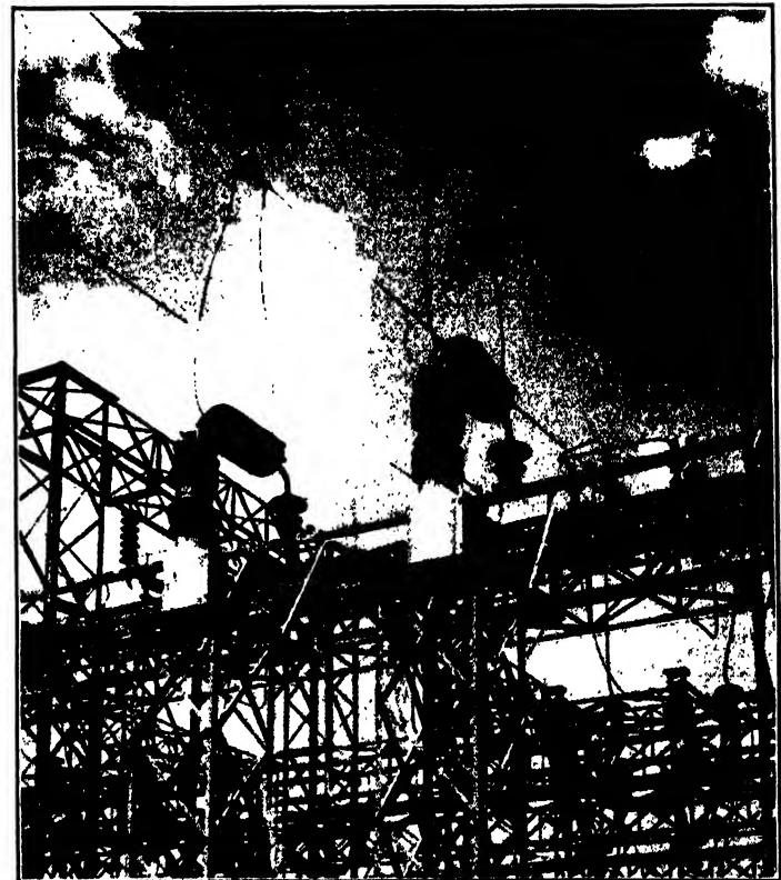
FIG. 25-18 Installation of line traps and coupling units in a substation structure.
