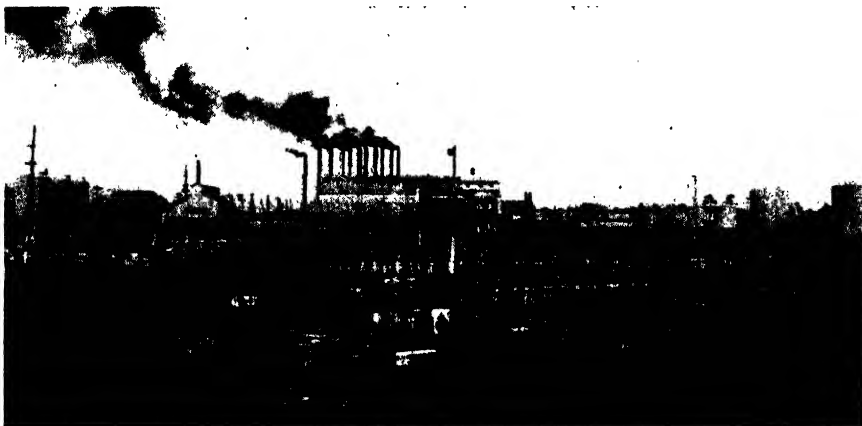
FIG. 11. Steam and Solvent Wood Rosin Plant.
